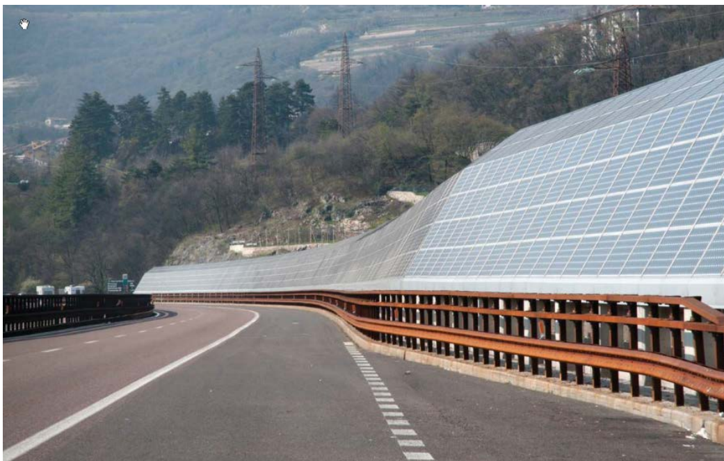
Figure 10: A photovoltaic noise barrier runs alongside the A22 autostrada at Brennero in Italy
