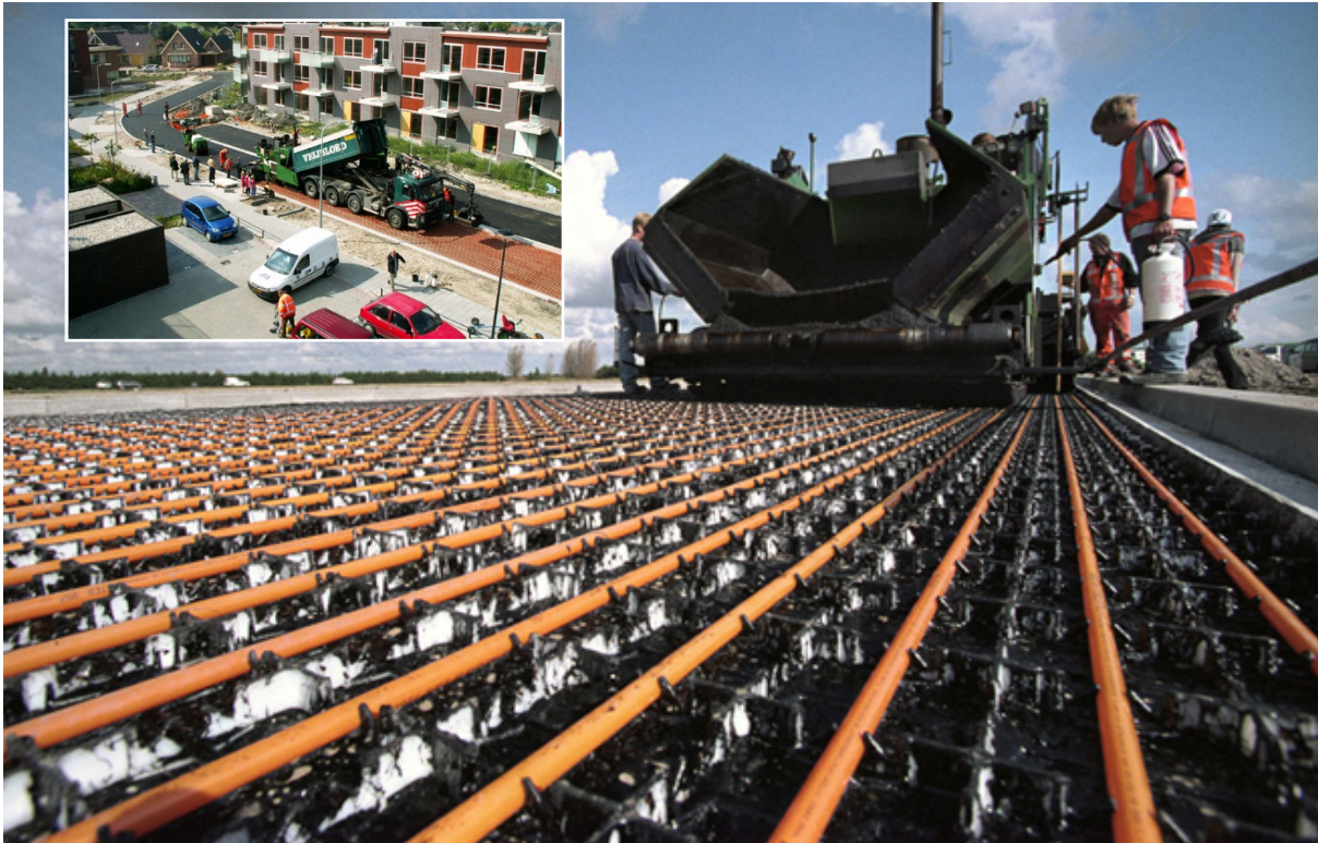
Figure 16: Water Cables Laid Under a Sheet of Asphalt
