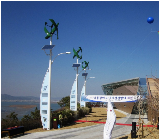
Figure 13: Examples of Hybrid Lamp Standards 80
