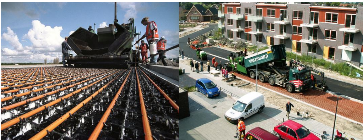
Figure 4: The use of pipework to extract heat from road surfaces for energy generation using aquifer heat exchangers in the Netherlands.
