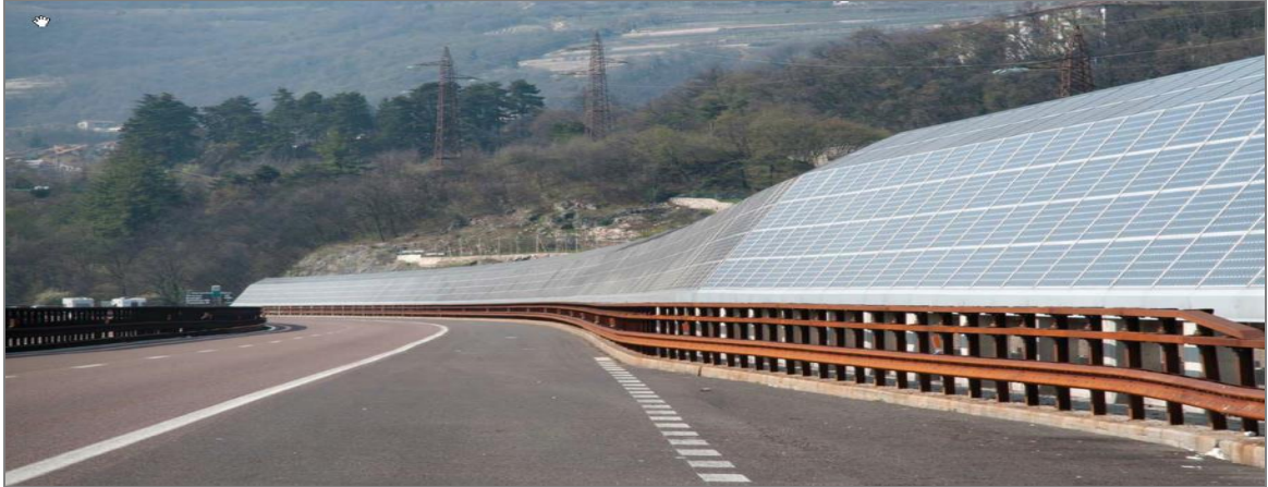
Figure 3: A photovoltaic noise barrier installed along the A22 Autostrada at Brennero in Italy.
