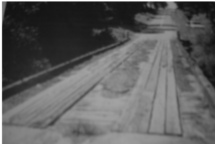
Figure 27.3 Weathered and Rotted Timber Deck of Bridge 1
