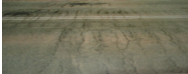
Figure 27.5 Bridge 2, Badly Cracked Wearing Surface Over One of the Piers
