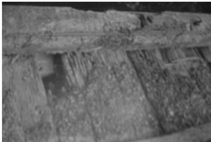
Figure 27.3 Weathered and Rotted Timber Deck of Bridge 1
