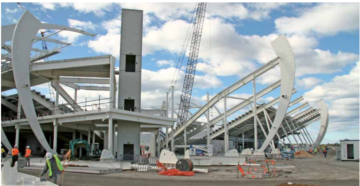
Off-site manufactured steel structures in place
