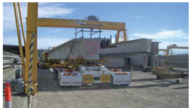
Jinkers being loaded with post-tensioned bridge beams
