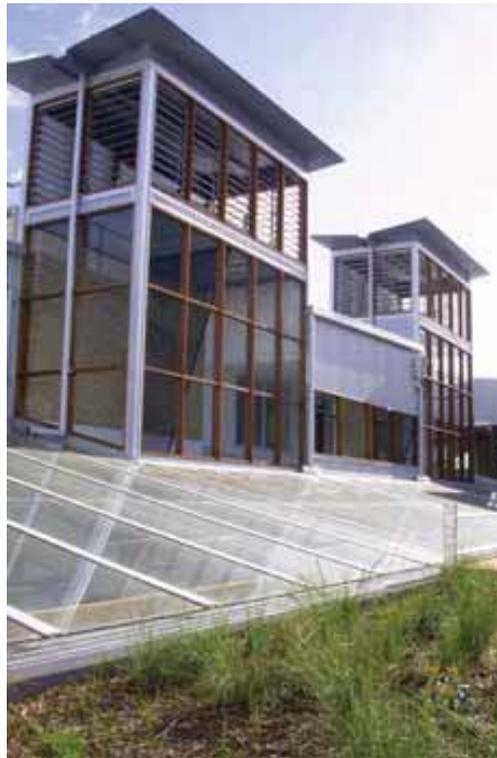
Figure 1: Thermal Chimneys<sup>26</sup>
